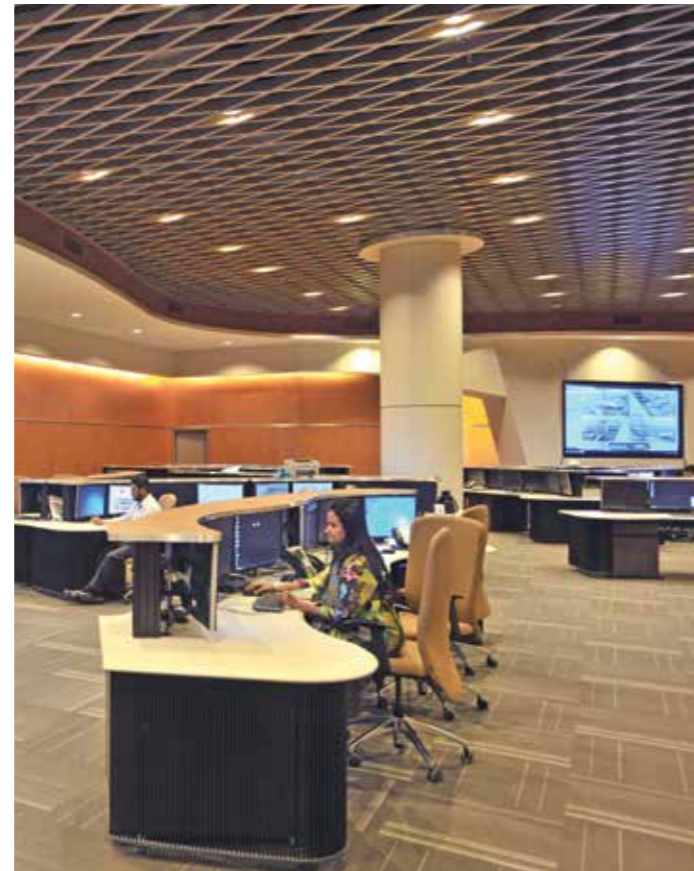
A state-of-the-art command and control centre at Mumbai International Airport
