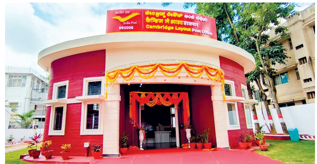
3D Concrete Printed Post Office Building, Bengaluru
