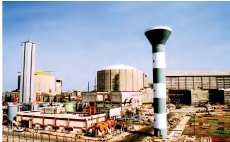
Tarapur atomic power plant
