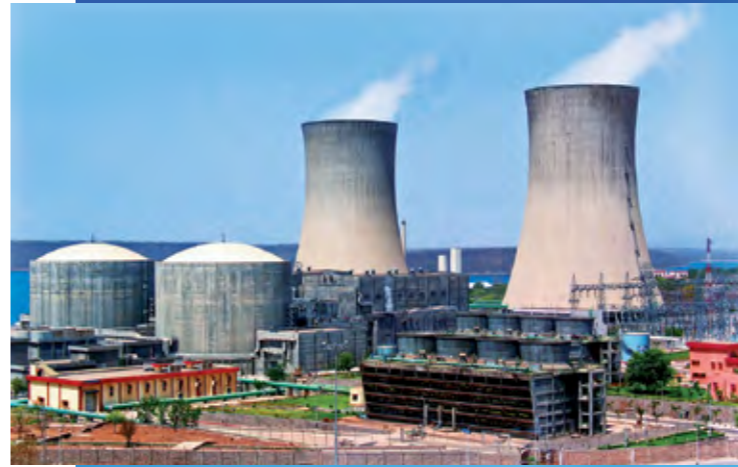
Rajasthan atomic power project
