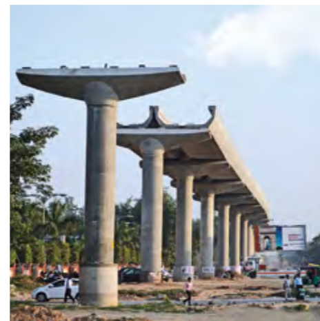
Precast 'U' girder for Delhi Metro
