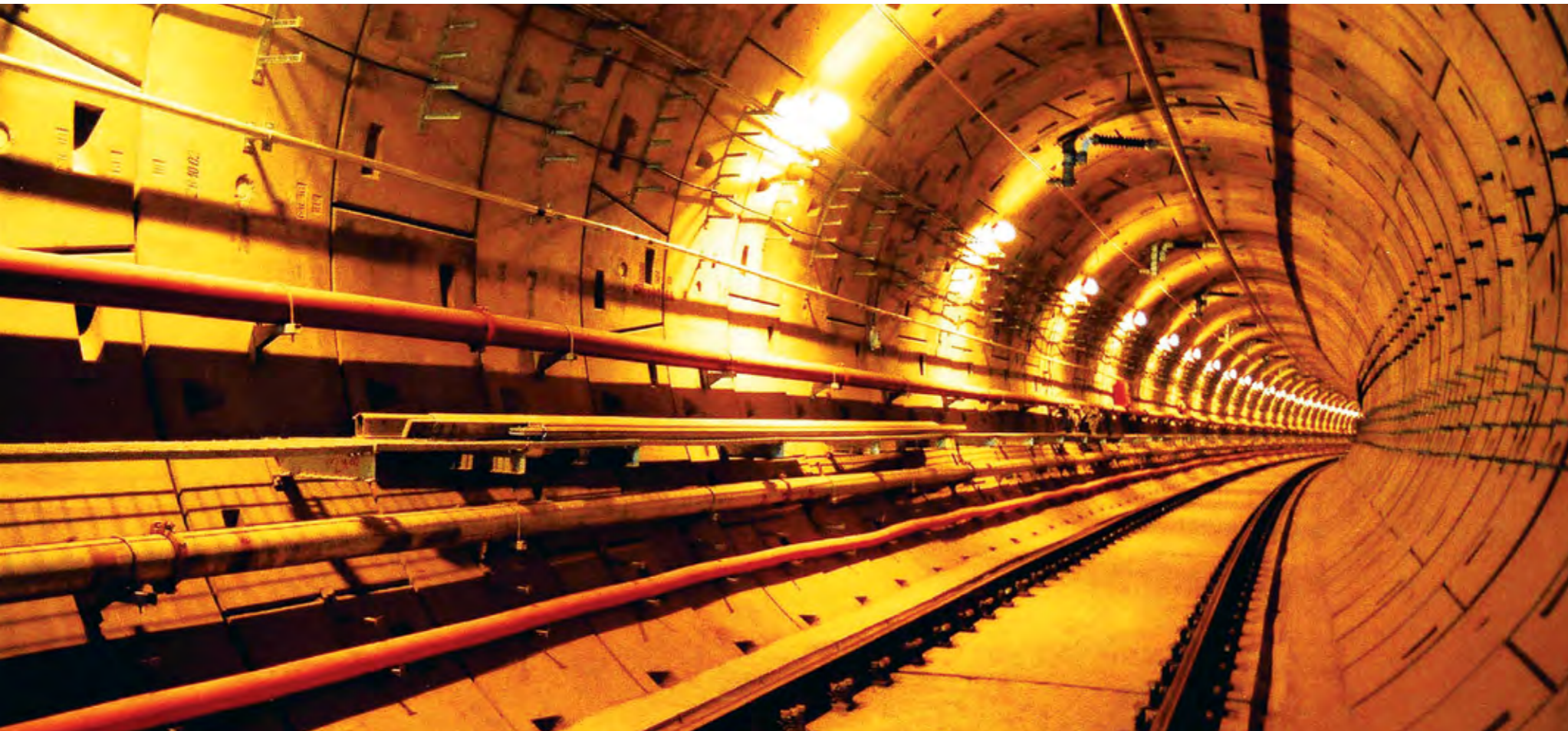
Underground section of Delhi Metro
