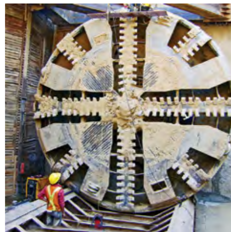
Tunnel Boring Machine
