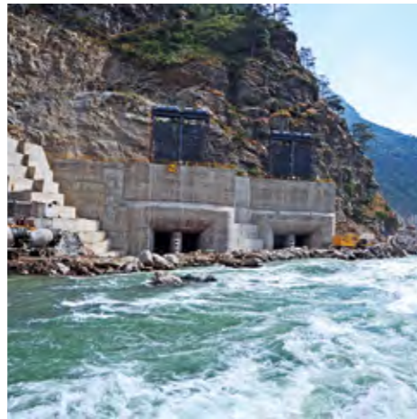
Intake structure at Punatsangchhu, Bhutan
