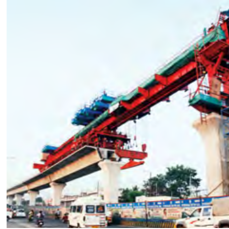
Girder erection for Hyderabad Metro
