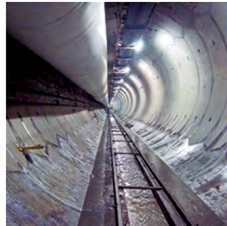
Head Race Tunnel, Tapovan Vishnugad
