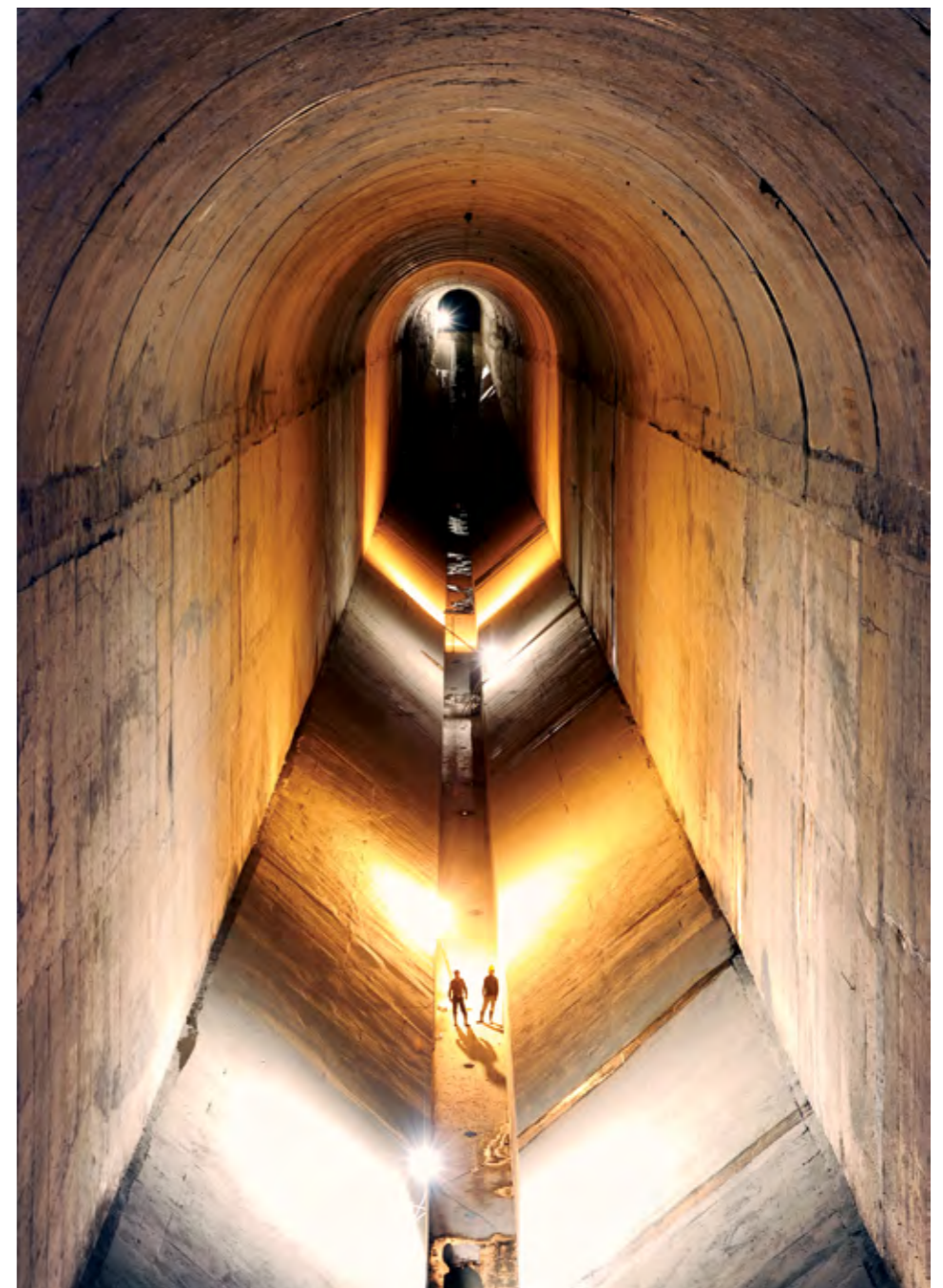
Underground desilting chamber, Parbati
