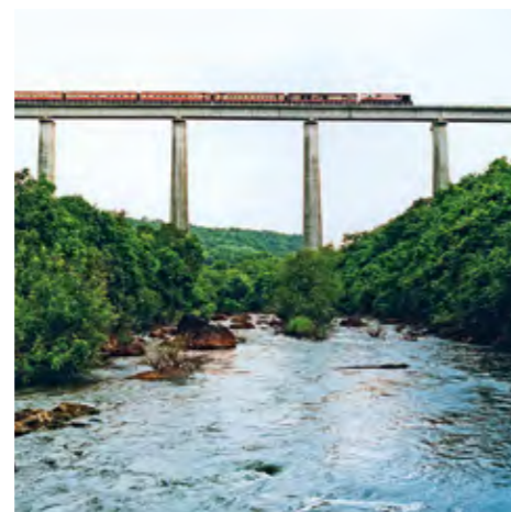
Panvel Nadi viaduct
