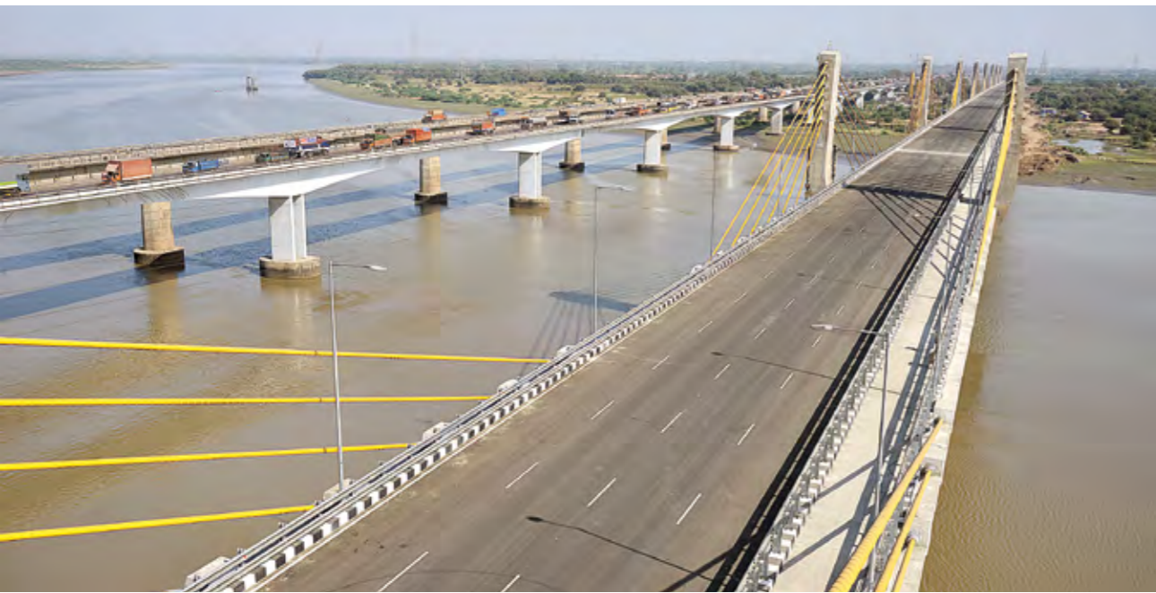
Arial view of third Narmada bridge
