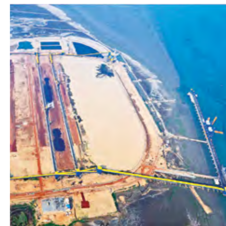
Dhamra port, Odisha
