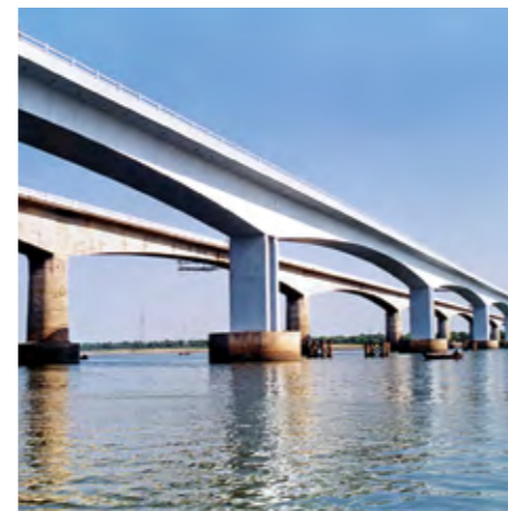
Second Narmada bridge, Gujarat
