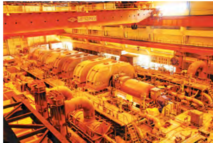
Turbine erection for Kudankulam nuclear power project
