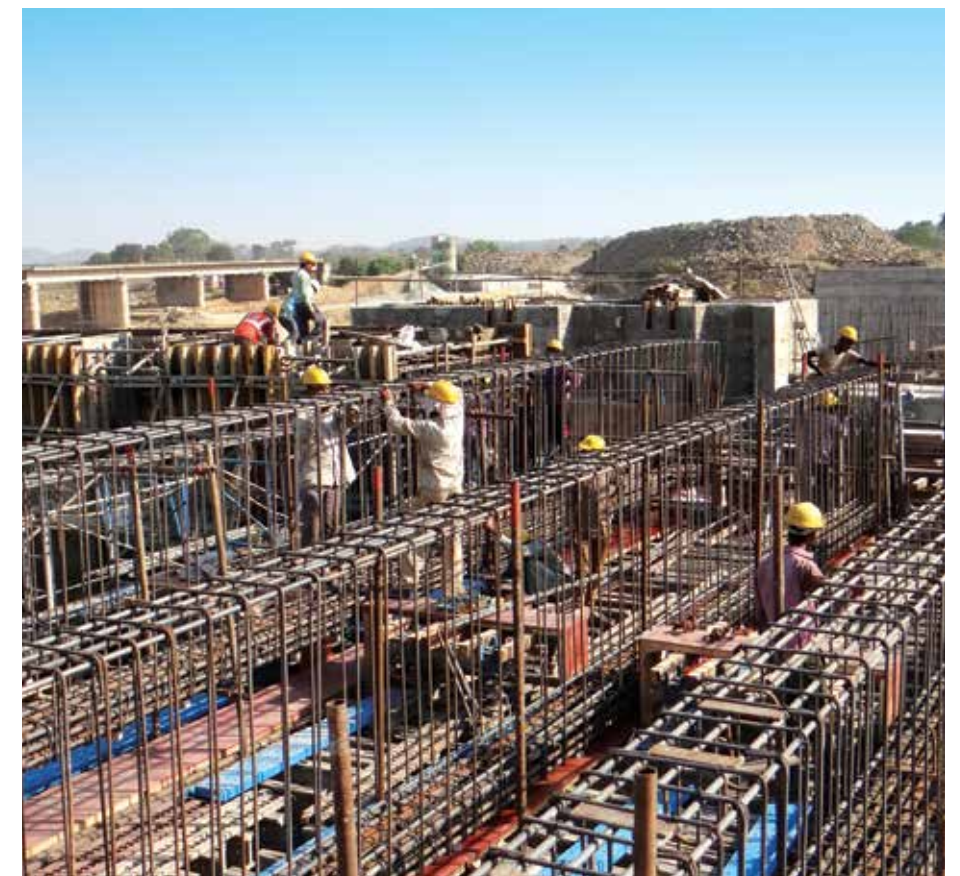
Reinforcement for deck slab
