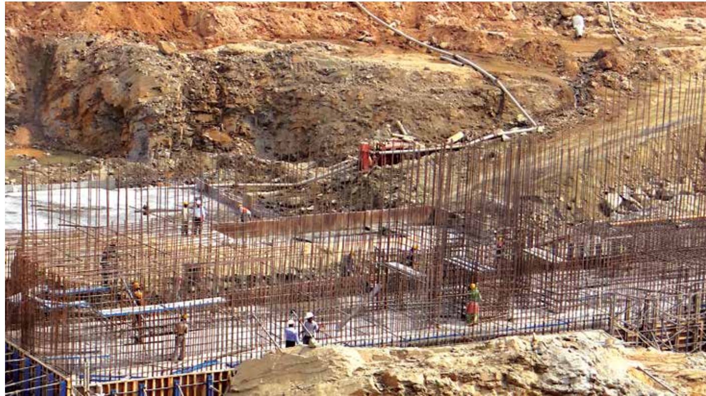
Reinforcement for pier footing
