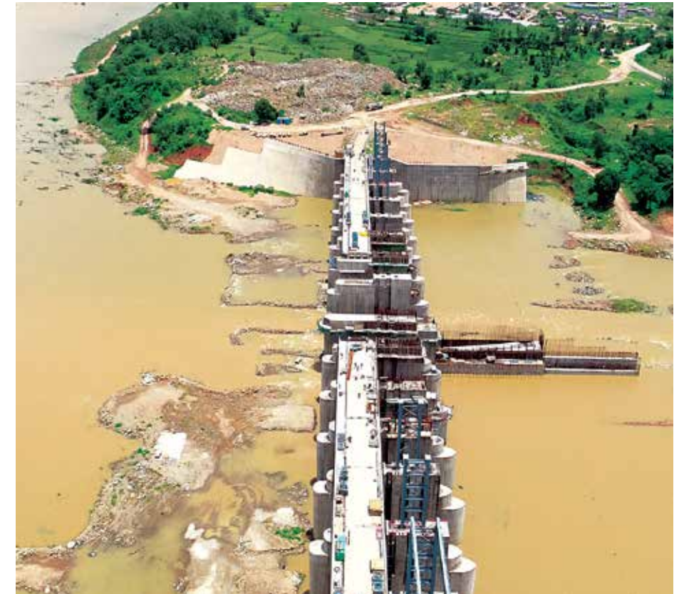
Aerial view of barrage
