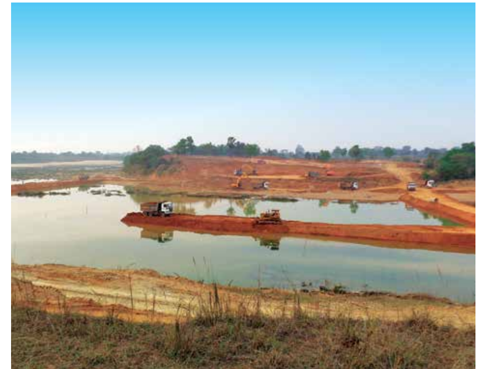
Coffer dam work in progress
