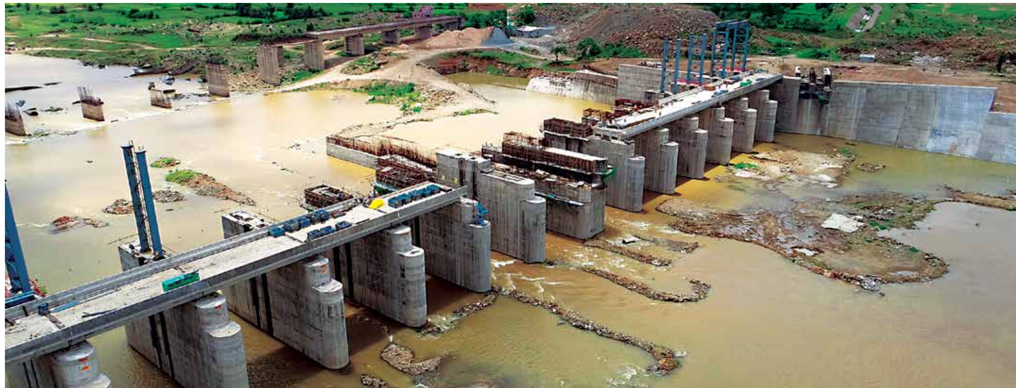
Right bank upstream view of Kharkai barrage
