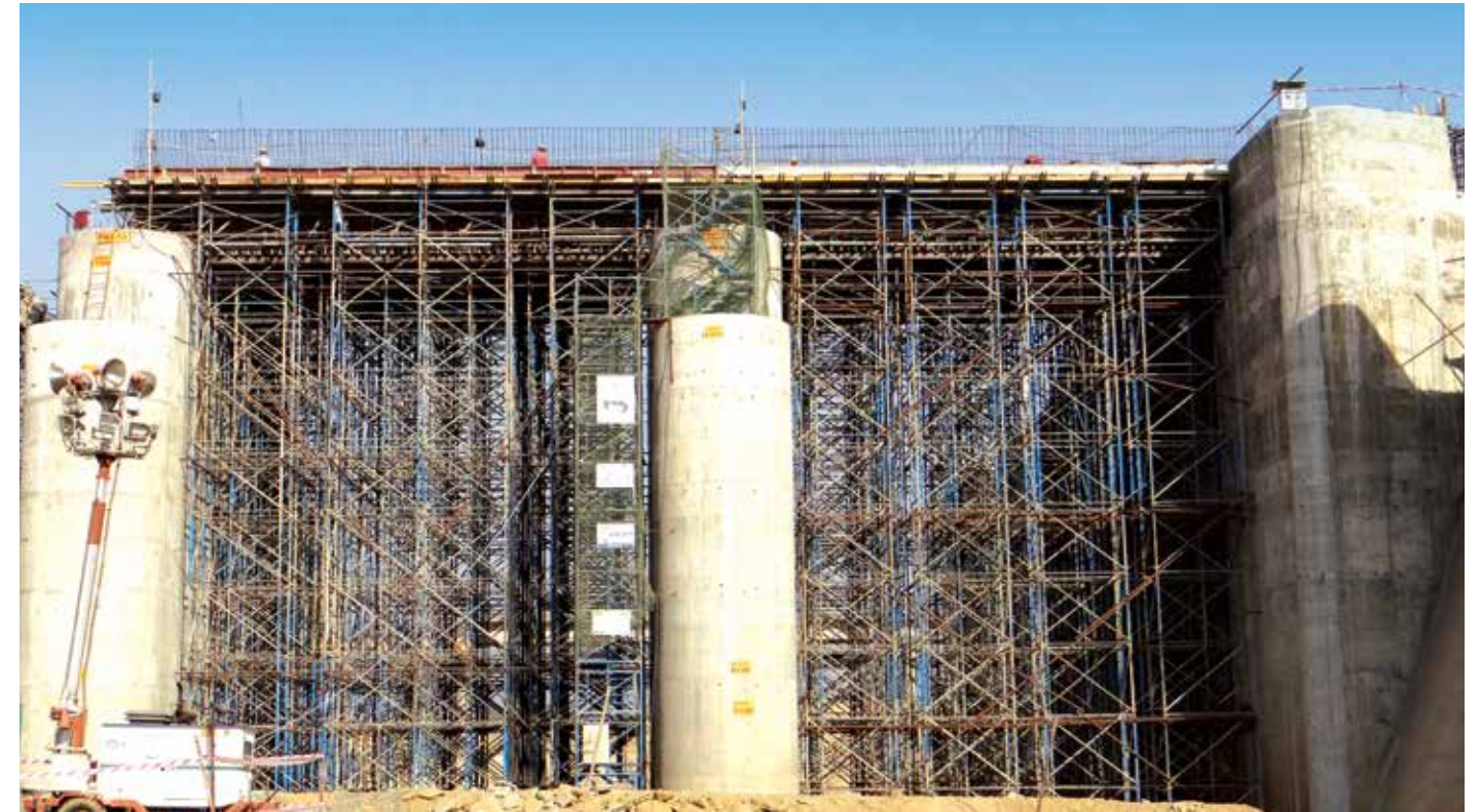
Staging for deck slab
