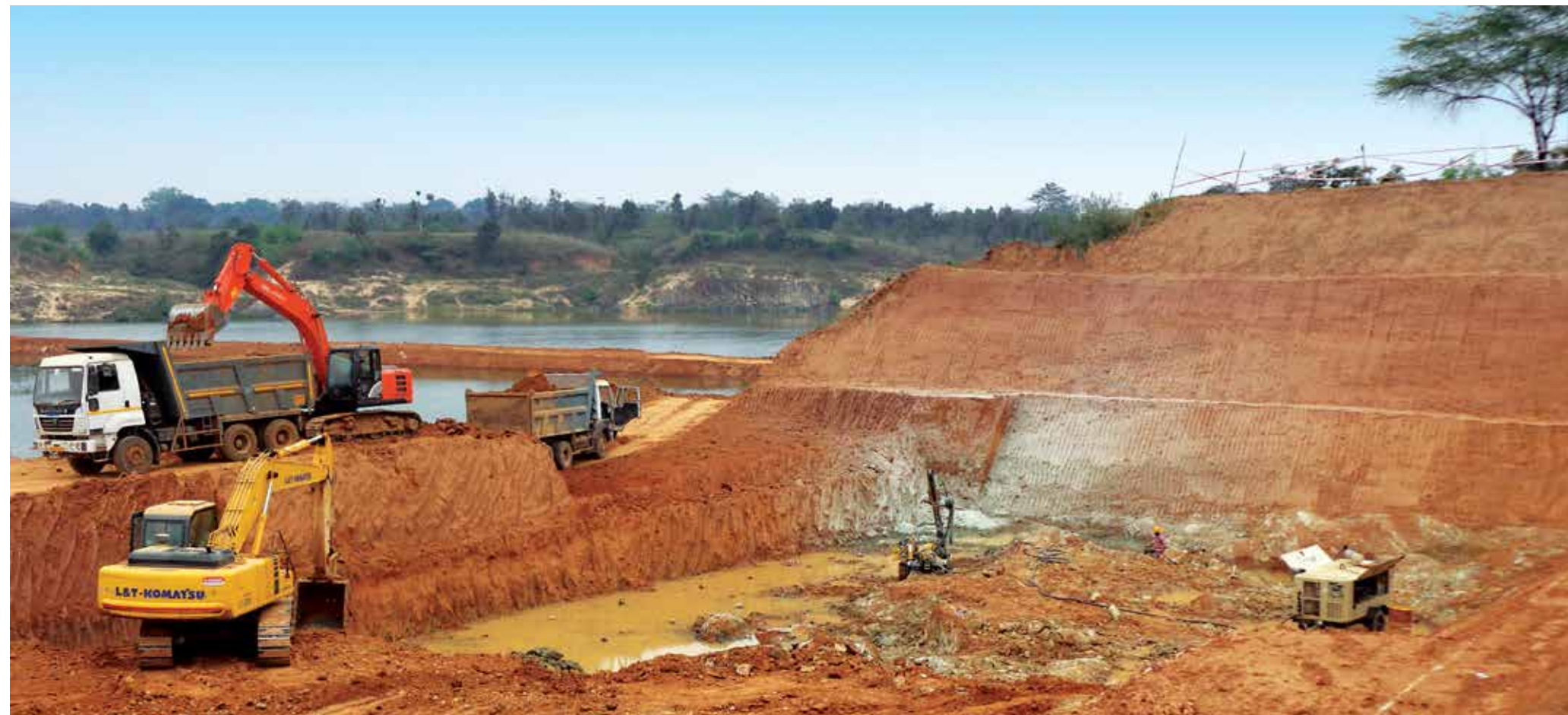
Excavation for left abutment
