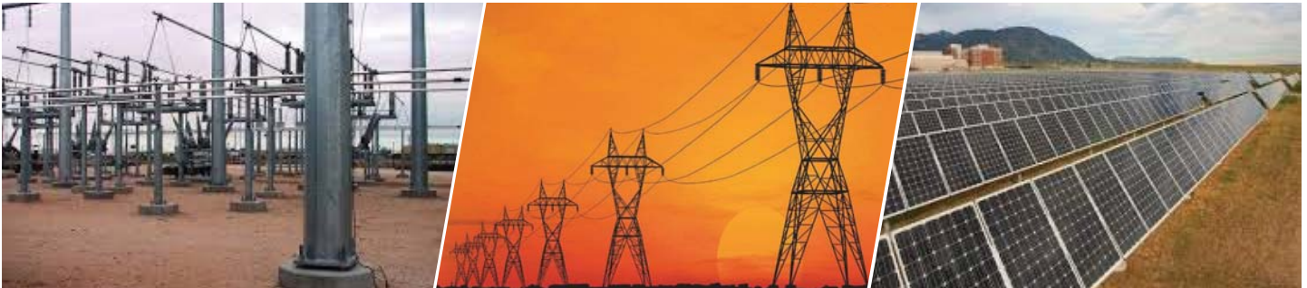
(Substation, Transmission Lines, Solar Farm)
