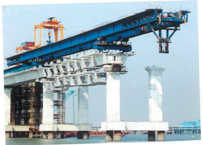
Fig.1: Marine Launching Girder during Load Test
