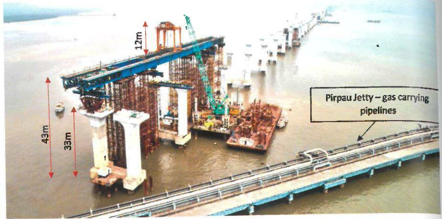
Fig. 4: Assembling of Launching Girder at 33 m Height near Pirpau Jetty
