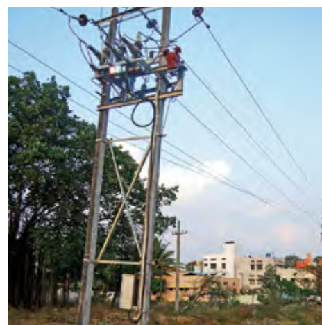
Auto recloser and sectionaliser works
