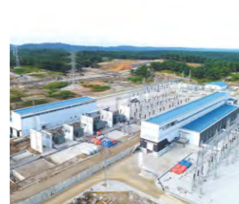
275/132/33 kV GIS at Samalaju in Malaysia
