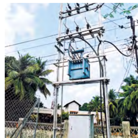
Power quality improvement works
