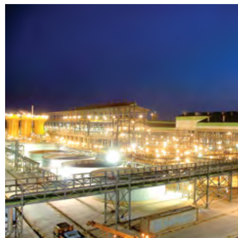
Electrification for a zinc plant
