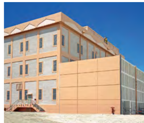
132/22 kV primary substation at Saadiyat Island in Abu Dhabi
