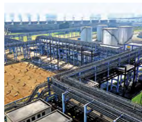
Cable tray installations at Jindal power plant
