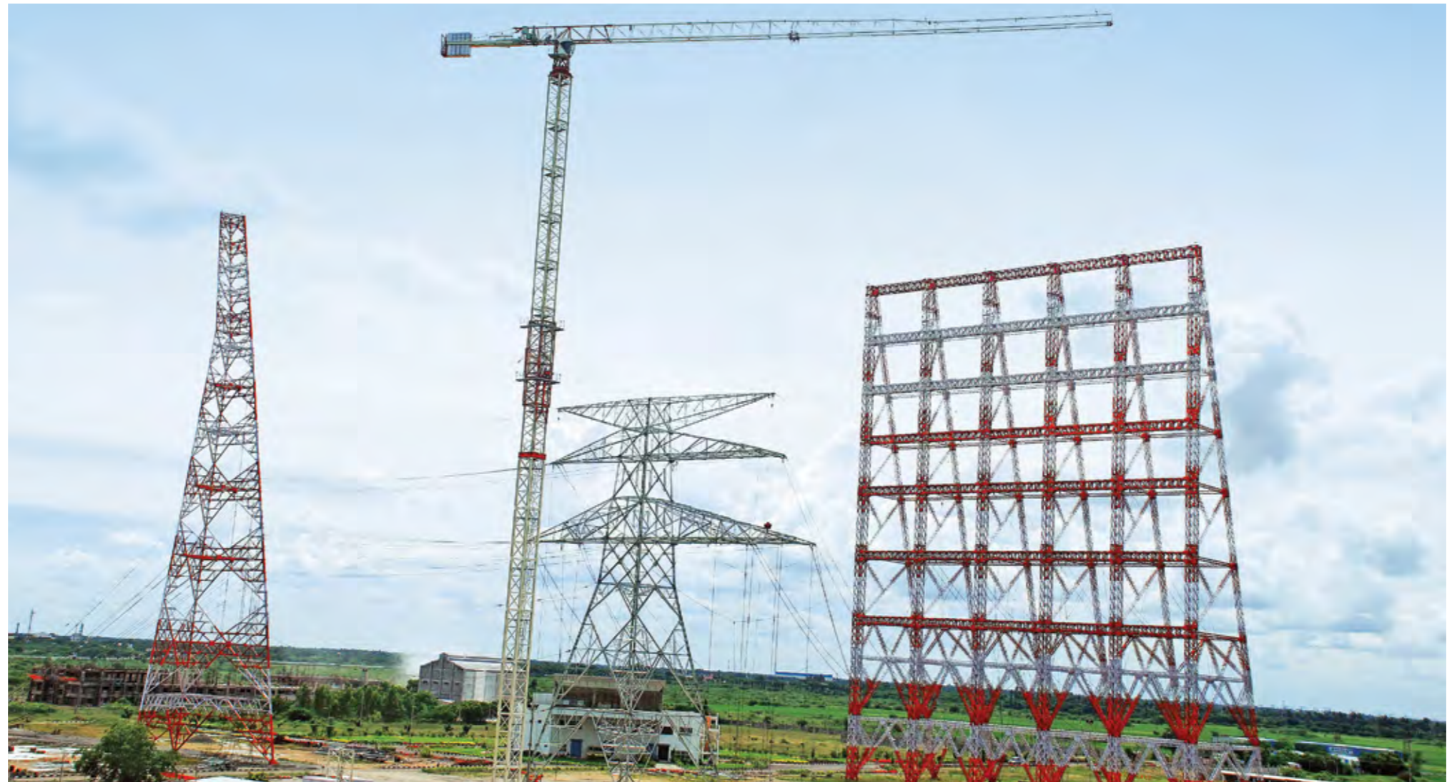
State-of-the-art tower testing station at Kancheepuram, near Chennai
