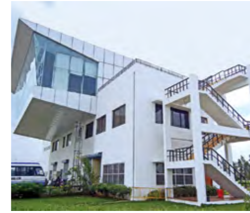
Control tower with a 360° view of the tower testing facility
