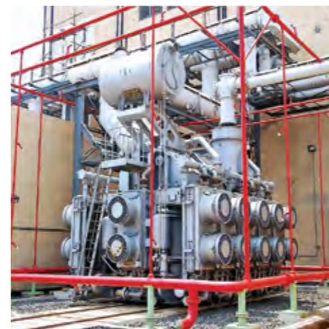
Installation and synchronization of transformer for a power plant
