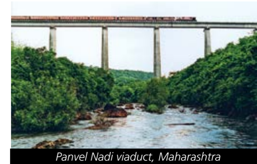
Panvel Nadi viaduct, Maharashtra
