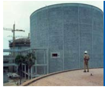
Reactor Building at Madras Atomic Power Plant, Kalpakkam
