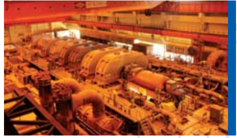
Turbine Erection for Kudankulam Nuclear Power Project
