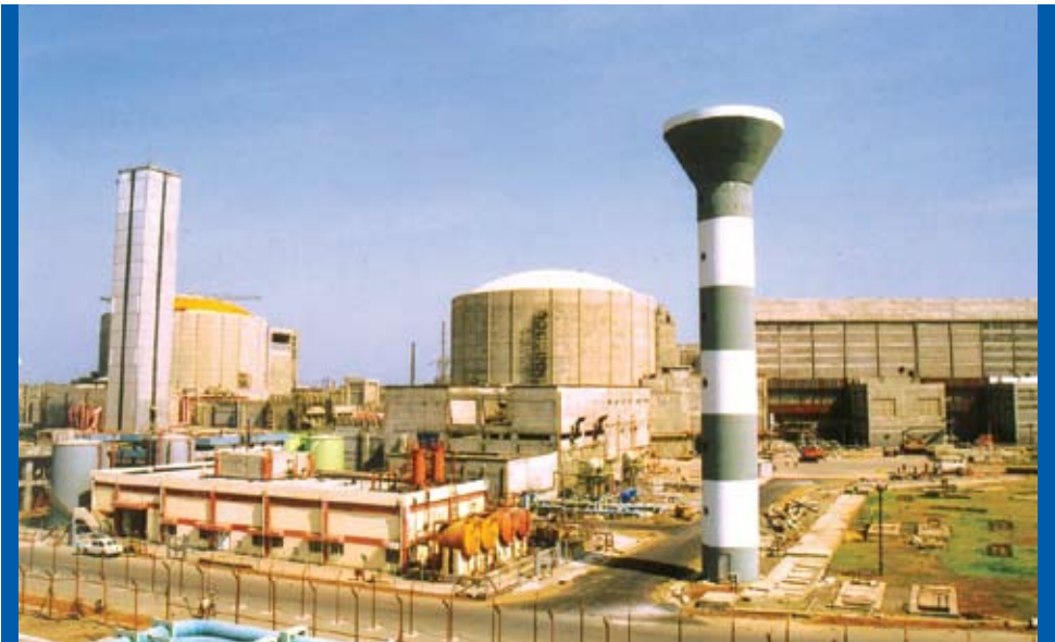
Unit 3 & 4 at Tarapur Atomic Power Project
