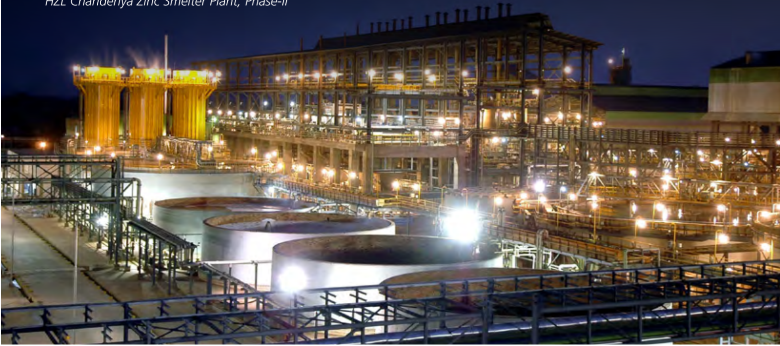
HZL Chanderiya Zinc Smelter Plant, Phase-II
