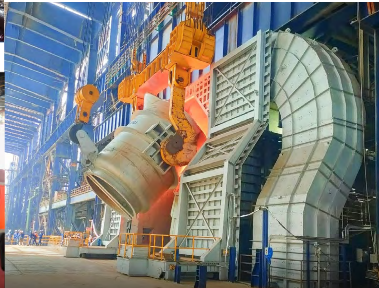
Steel Melt Shop #2 - 350 t Converter 1 at JSW Dolvi
