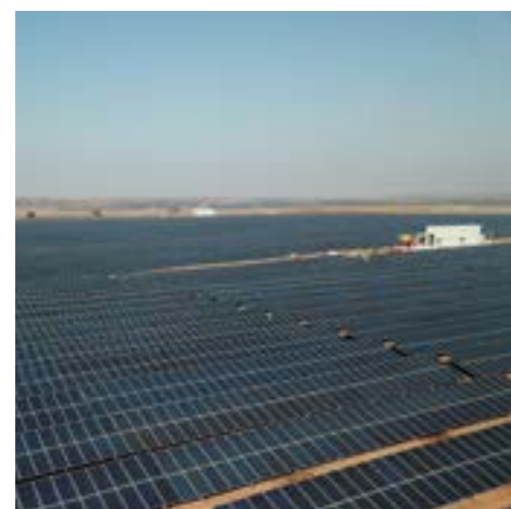
324 MWp Fixed Tilt Solar PV Project at Rewa Ultra Mega Solar Park (RUMS), Madhya Pradesh
