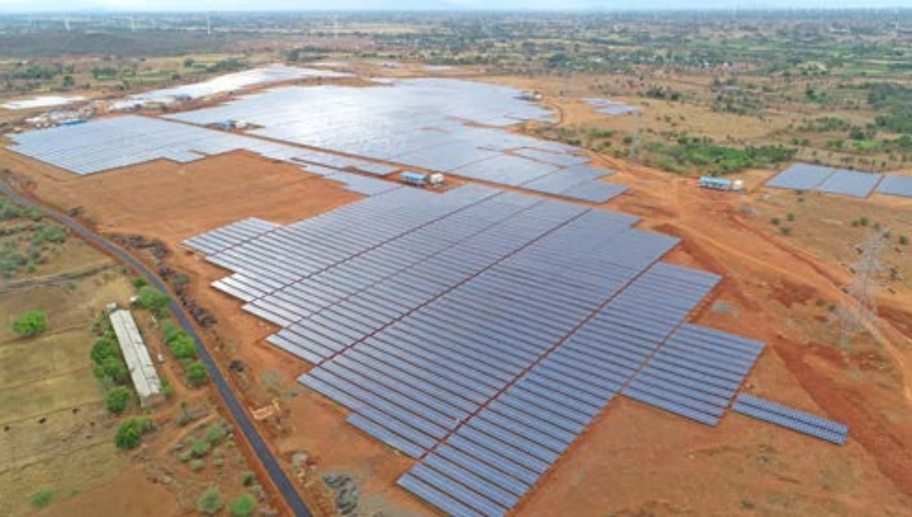
Work in Progress at a Solar PV Plant
