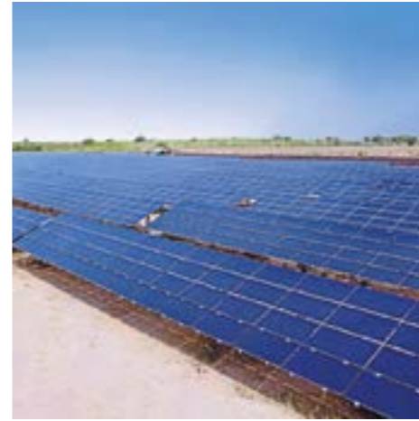
Thin film A-Si technology
