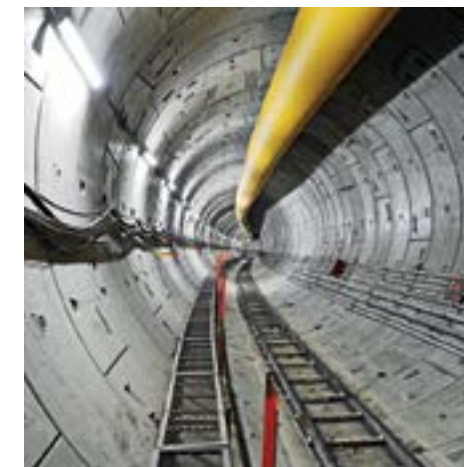
Underground section of Chennai Metro
