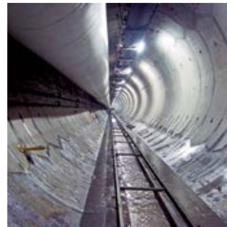
Head Race Tunnel, Tapovan Vishnugad
