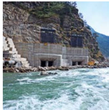
Intake structure at Punatsangchhu, Bhutan
