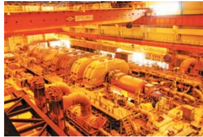
Turbine erection for Kudankulam nuclear power project
