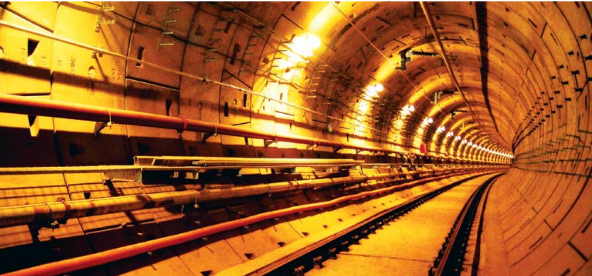
Underground section of Delhi Metro
