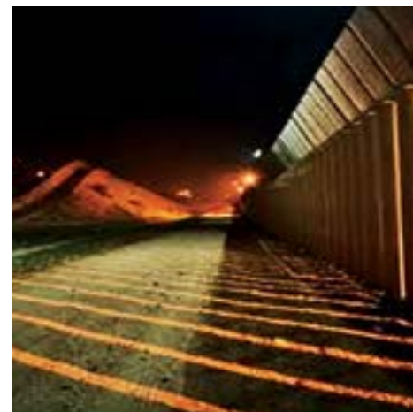
Blast walls / fences
