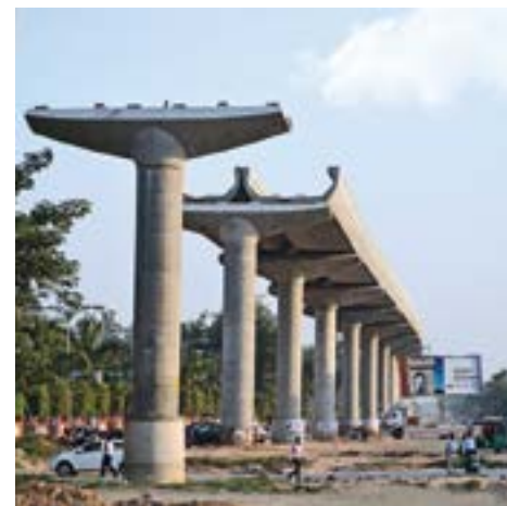
Precast 'U' girder for Delhi Metro
