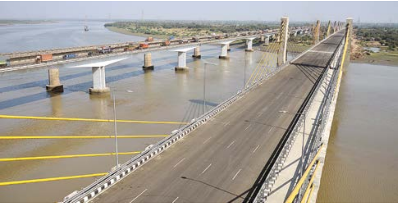
Arial view of third Narmada bridge
