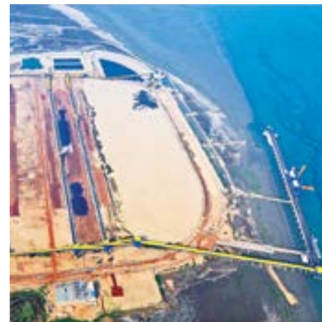
Dhamra port, Odisha
