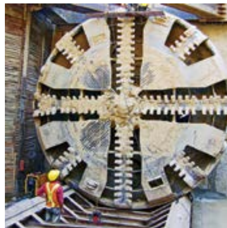
Tunnel Boring Machine
