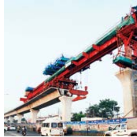
Girder erection for Hyderabad Metro
