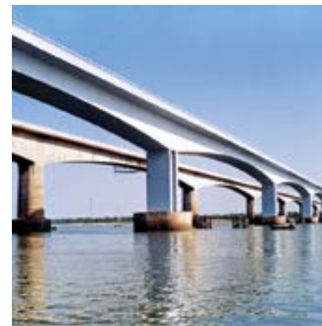
Second Narmada bridge, Gujarat
