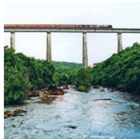
Panvel Nadi viaduct
