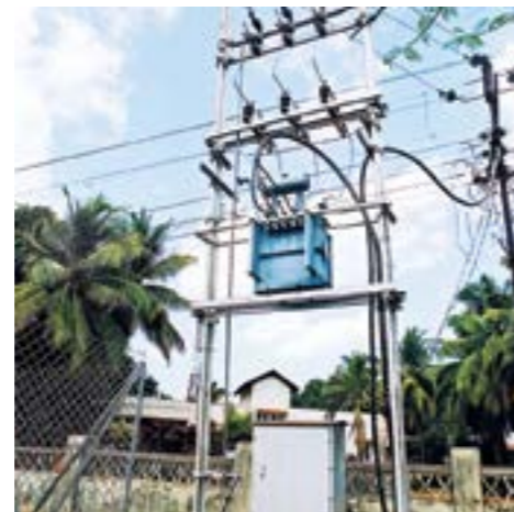
Power quality improvement works
