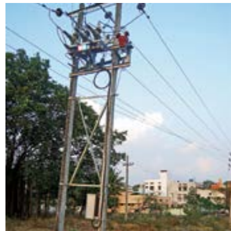
Auto recloser and sectionaliser works
