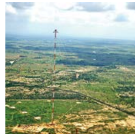
471 m high guyed mast communication tower - the tallest in India
