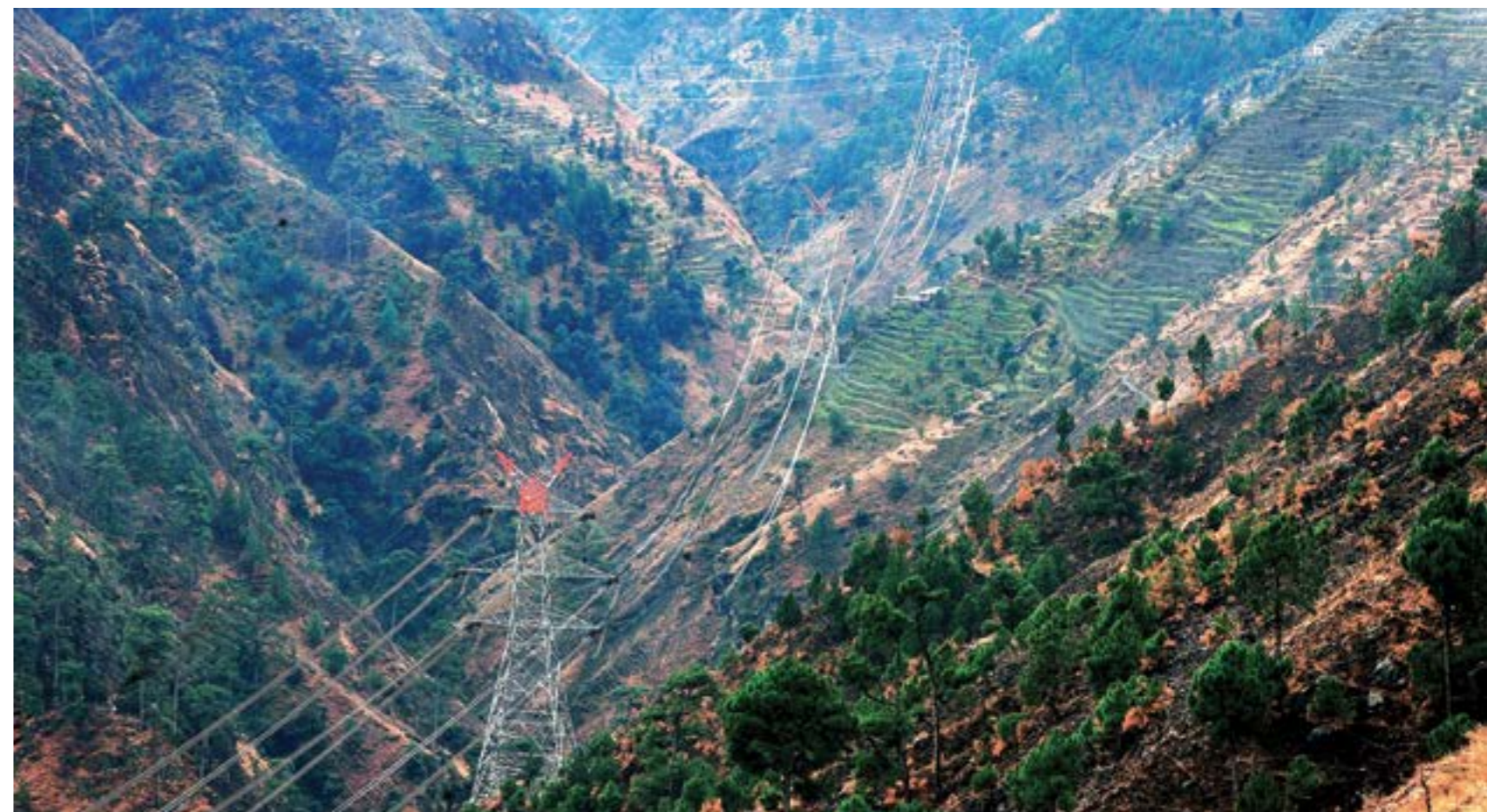
400 kV double circuit Karcham Wangtoo - Abdullapur transmission line
