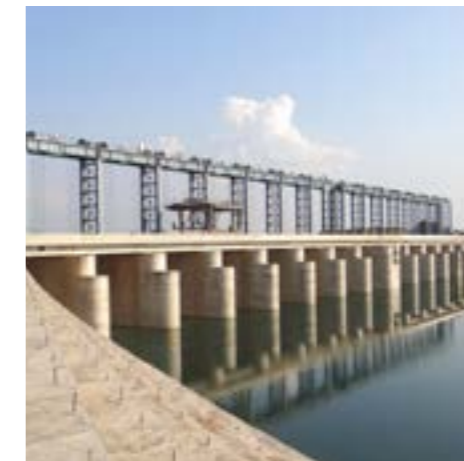
Kharkai Barrage, Jharkhand
