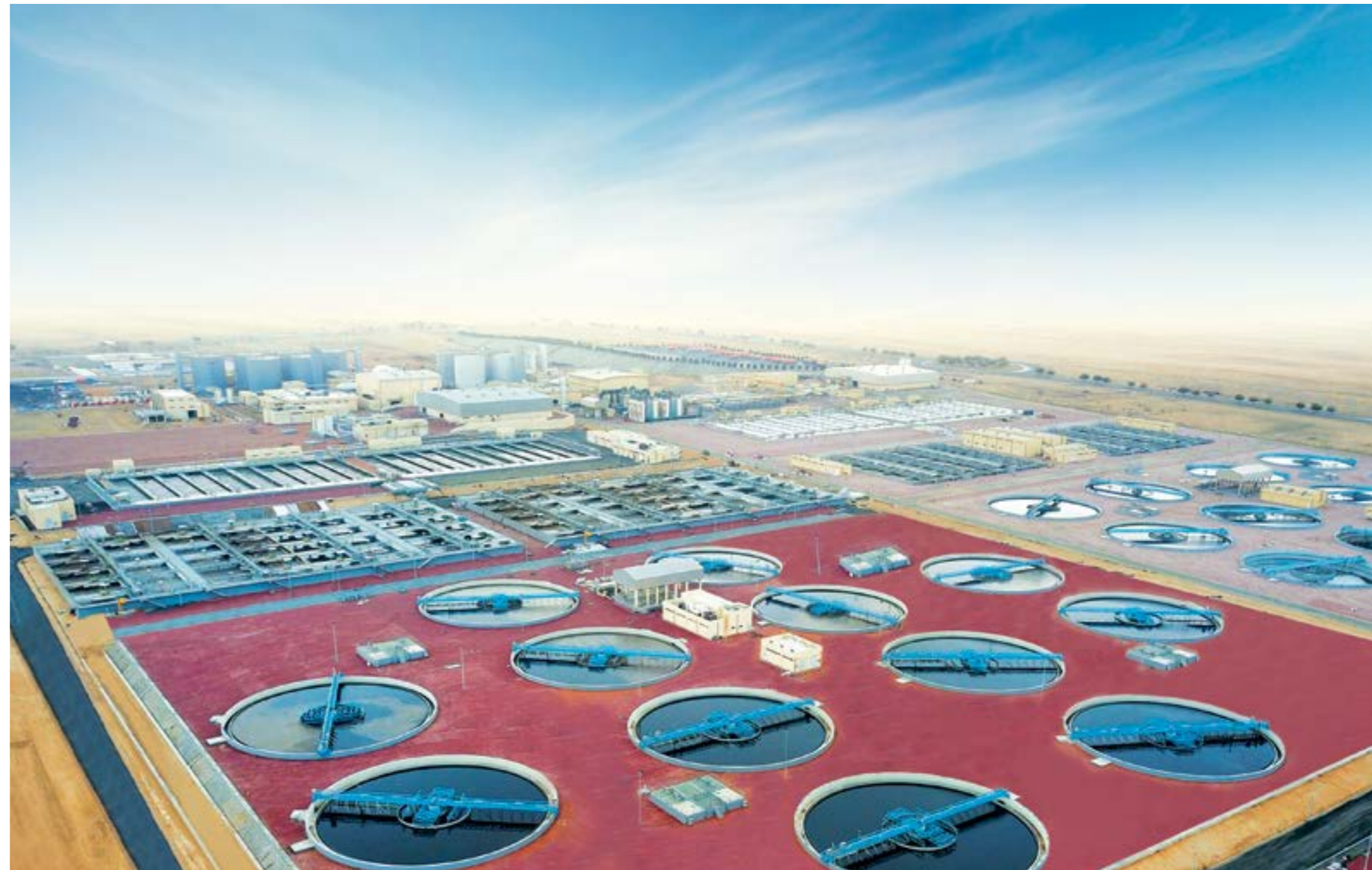
375 MLD Wastewater Treatment Plant, Jebel Ali, UAE
