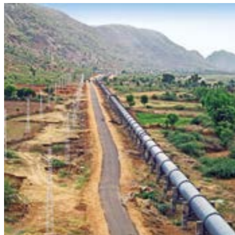
Transmission Mains, Bisalpur, Rajasthan
