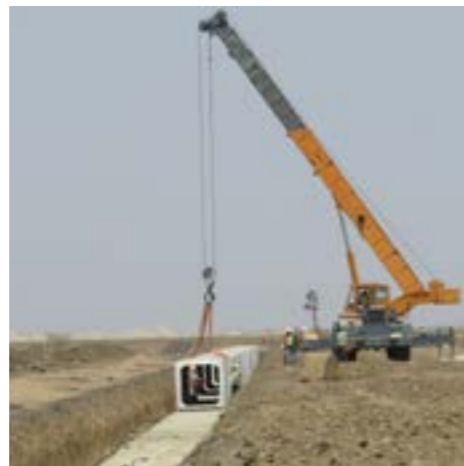
Precast duct laying at Amaravati, Andhra Pradesh
