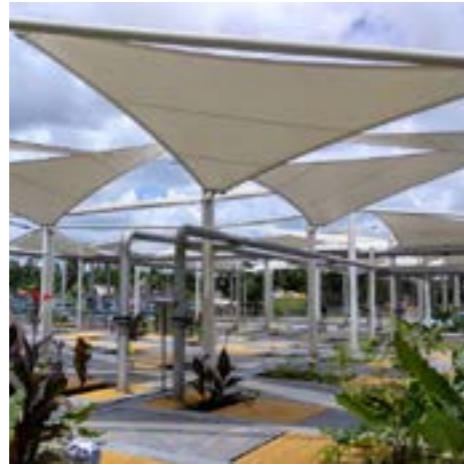
31 MLD Wastewater Treatment Plant, Bhatpara, West Bengal
