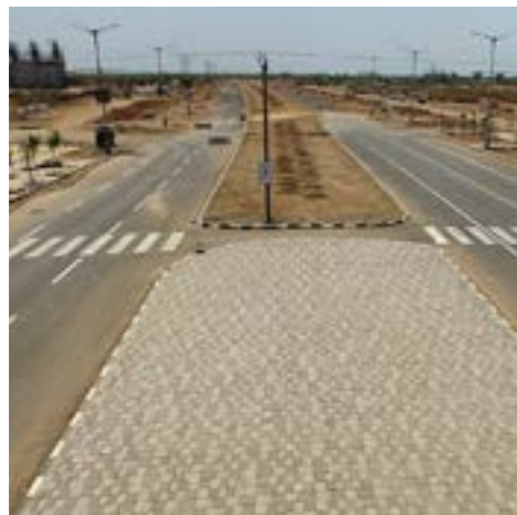
Green-field development at Dholera, Gujarat
