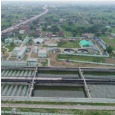
120 MLD Wastewater Treatment Plant, Varanasi, Uttar Pradesh
