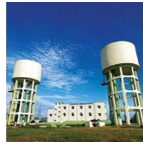
Ali Sagar Lift Irrigation Scheme, Telangana
