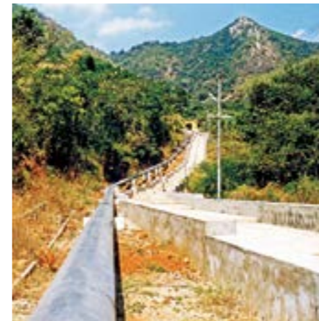
Pipeline installed on steep gradients
