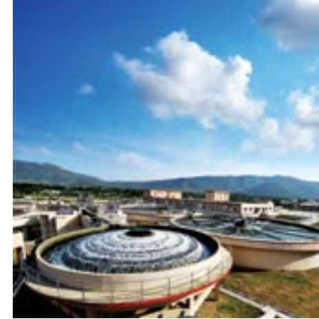
181 MLD Water Treatment Plant, Vellore, Tamil Nadu
