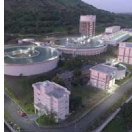
137 MLD Water Treatment Plant at Nashik, Maharashtra
