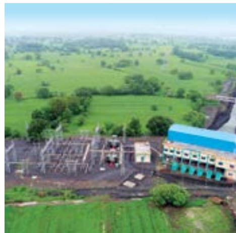
Mohanpura Lift Irrigation Project, Madhya Pradesh
