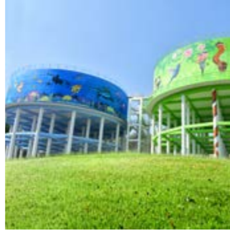
Elevated Storage Reservoir, Pune, Maharashtra
