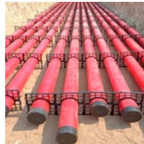
PLB Duct at Amaravati, Andhra Pradesh
