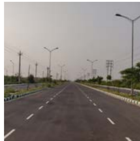
Integrated infrastructure development, Rohtak, Haryana
