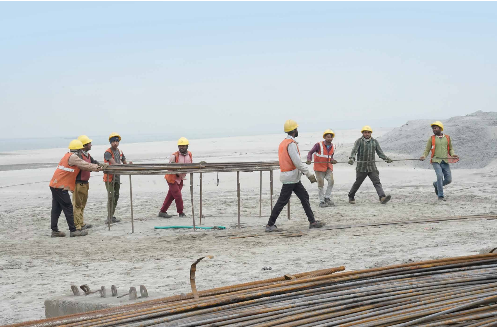
L&T workmen busy bar-bending at Birsing island.
