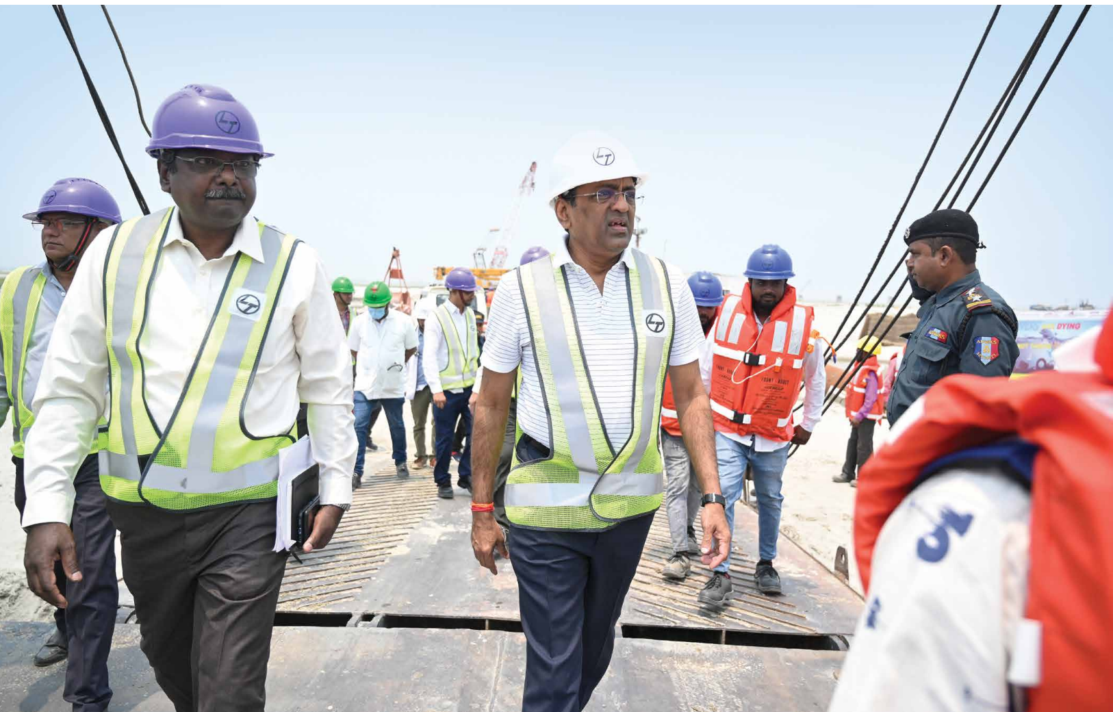
L&T CMD Mr S N Subrahmanyam (right) with Project Director Mr V R Saravanakumar during a visit to the bridge site in 2023.
