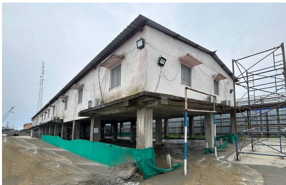
To avert flooding, the L&T project office at Phulbari sits on stilts.
