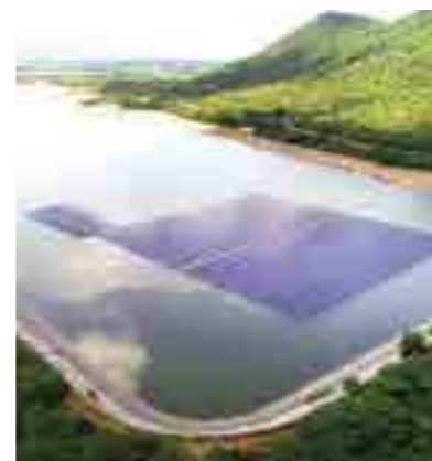
4 MWp Floating Solar PV Project, Tirupati
