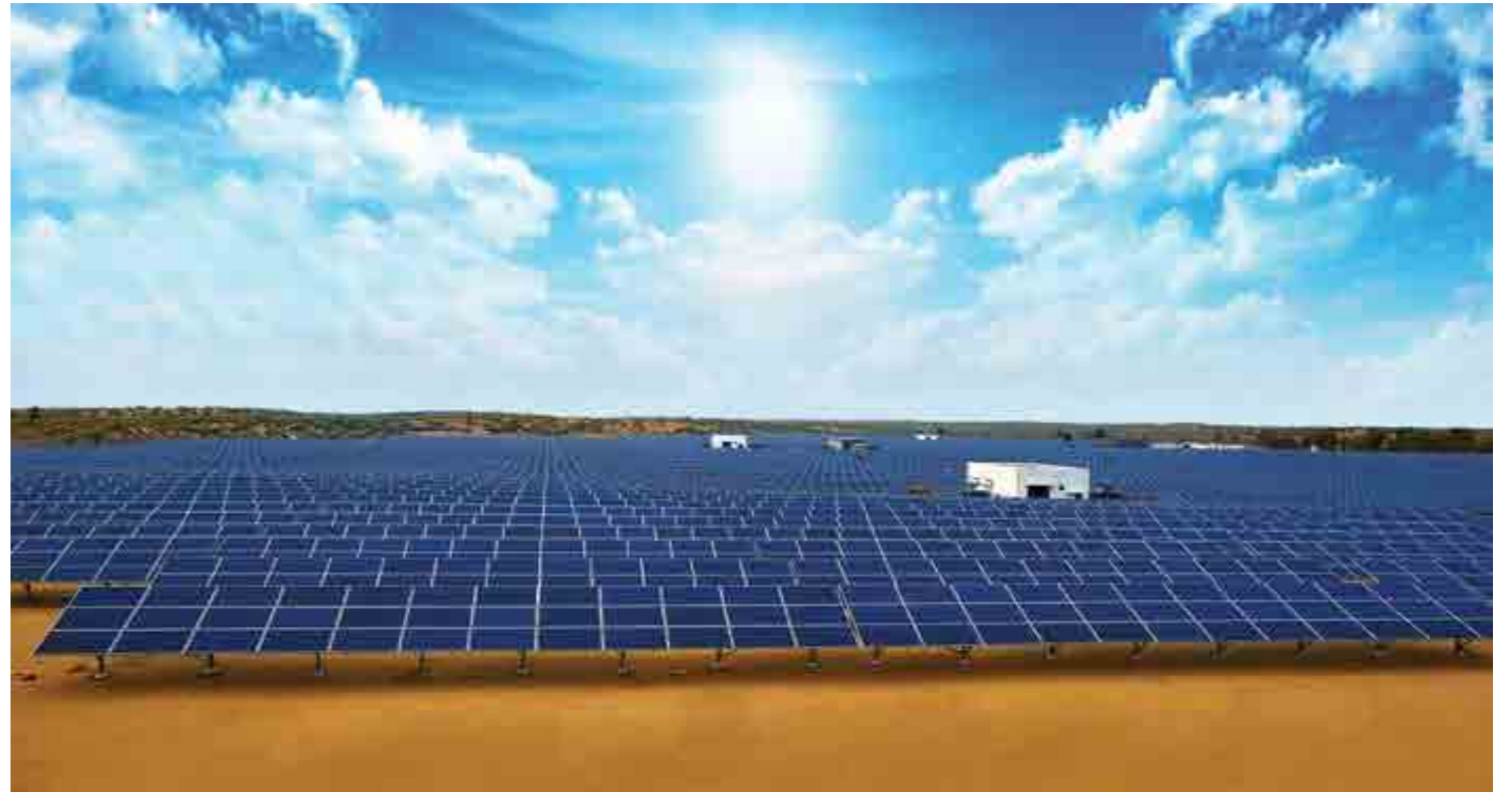
22 MWp Solar PV Power Plant at Rajasthan
