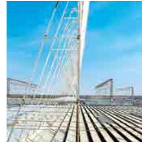
Asia's largest CSP plant 125 MWe solar thermal power plant (600 acres) at Pokhran, Rajasthan
