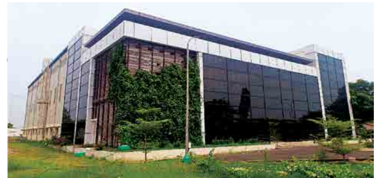
Container Integration Facility - L&T, Kanchipuram
