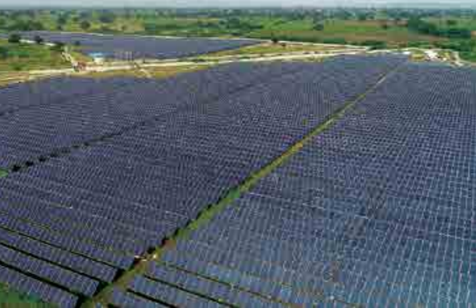
209 MWp/190 MW Solar Tracker Project, Karnataka
