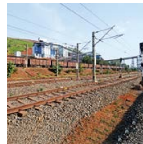
Dedicated track for a steel plant
