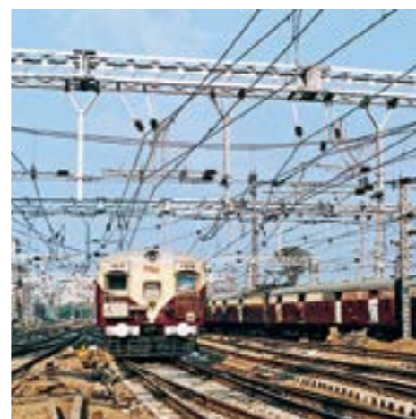
Portal corridors at Mumbai CST yard
