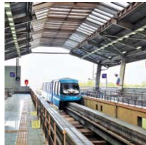
Mumbai Monorail station building
