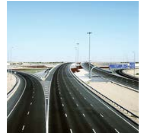
Sheikh Khalifa interchange, connecting Dubai and Abu Dhabi
