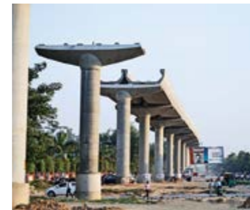
Full span 'U' girder for Delhi Metro
