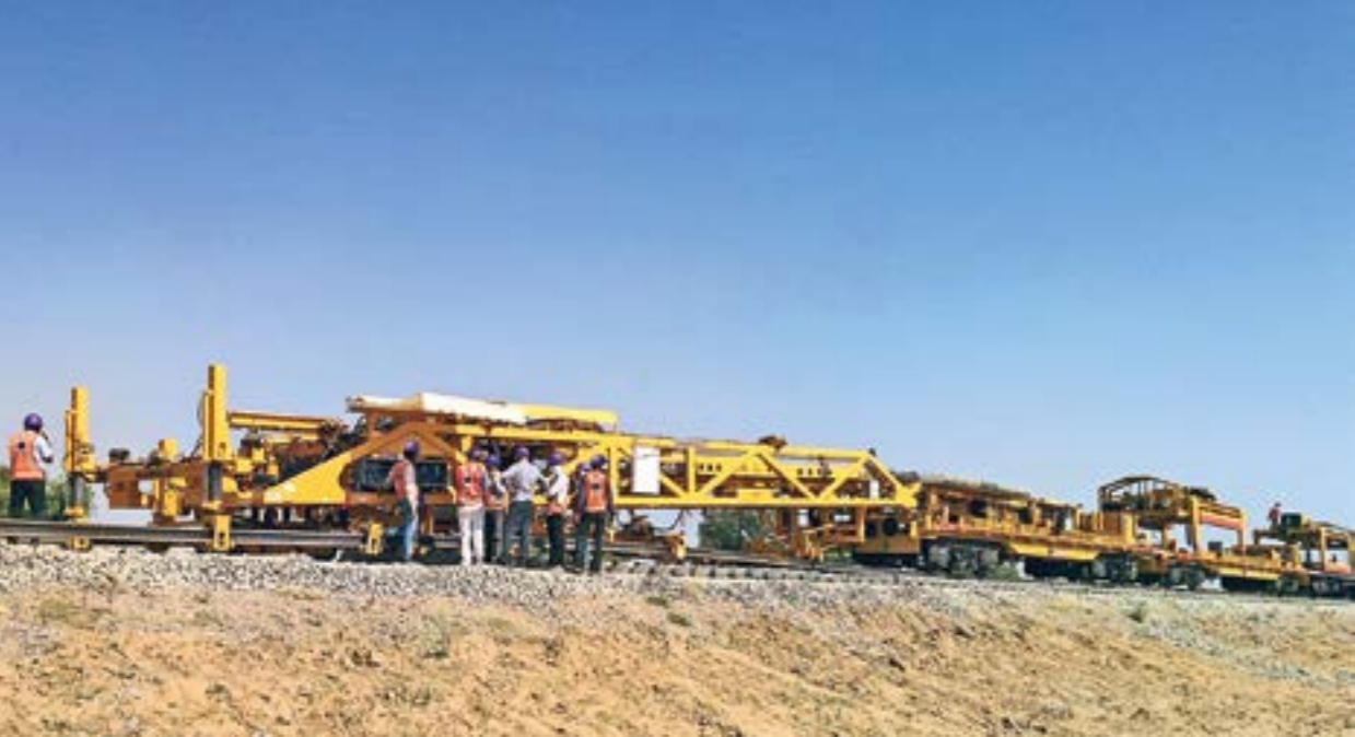
Mechanized track laying
