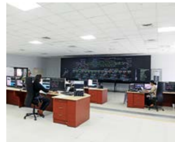
Operations and command centre of Mumbai Monorail
