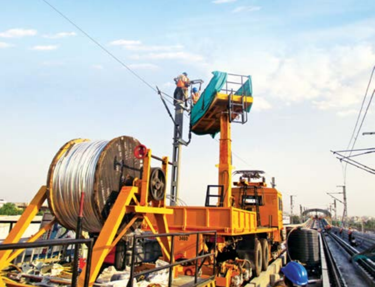
Railway electrification works
