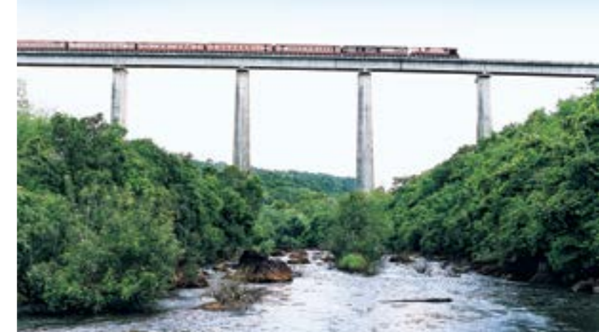
Panvel Nadi viaduct
