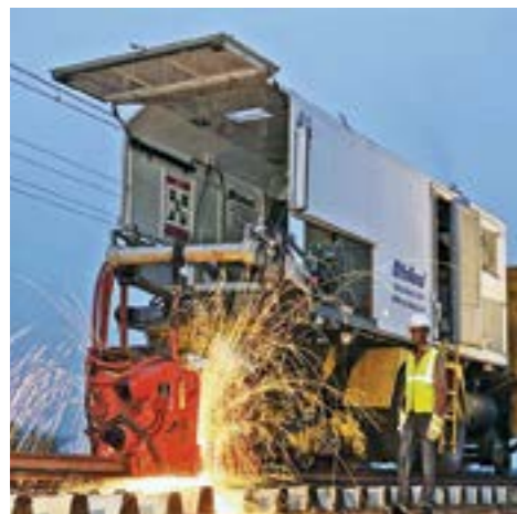
Flash butt welding
