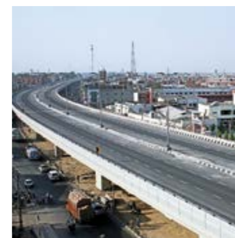
Panipat elevated corridor
