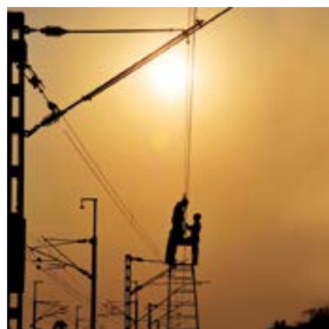
Electrification of the Tiruvallur - Arakonam section
