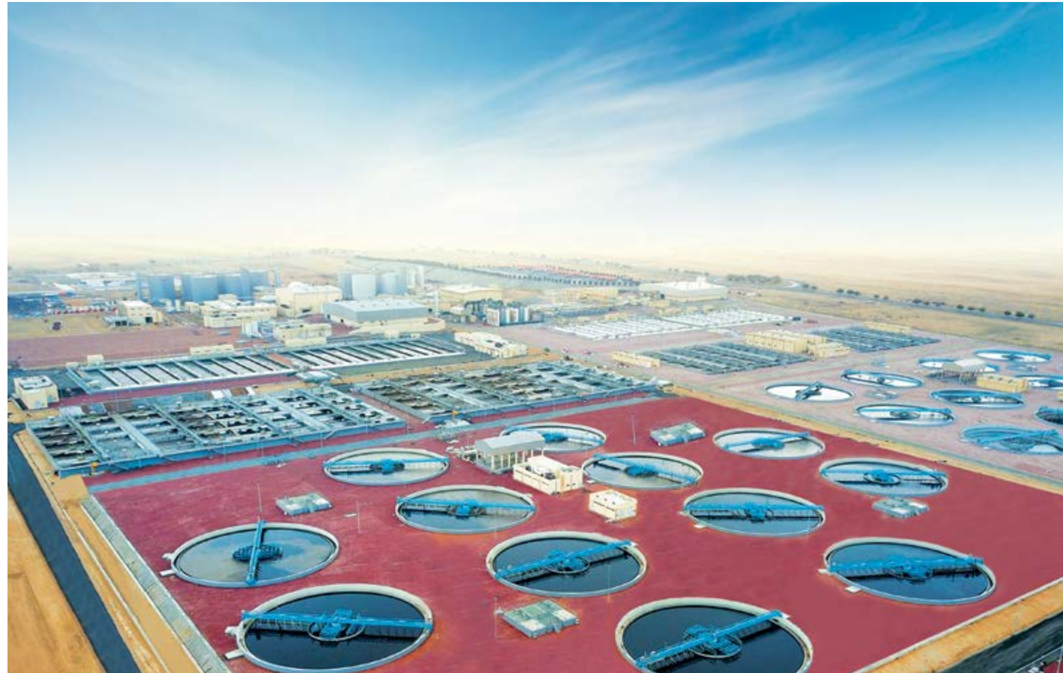
375 MLD Wastewater Treatment Plant, Jebel Ali, UAE
