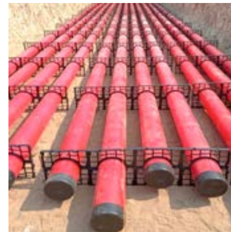
PLB Duct at Amaravati, Andhra Pradesh
