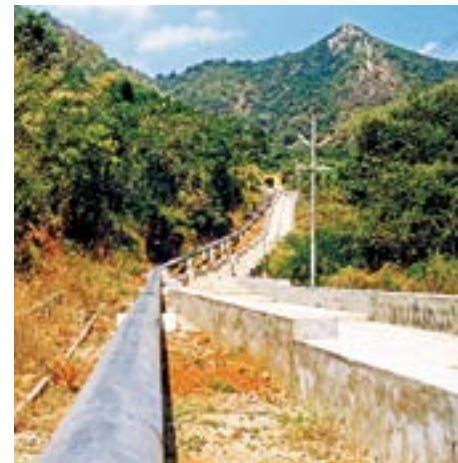
Pipeline installed on steep gradients
