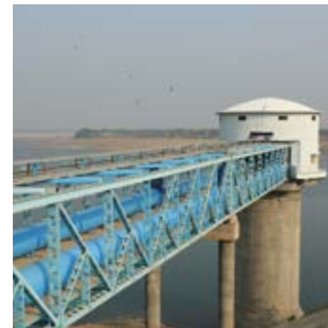
Lift Irrigation Scheme for GIDC at Dahej, Gujarat
