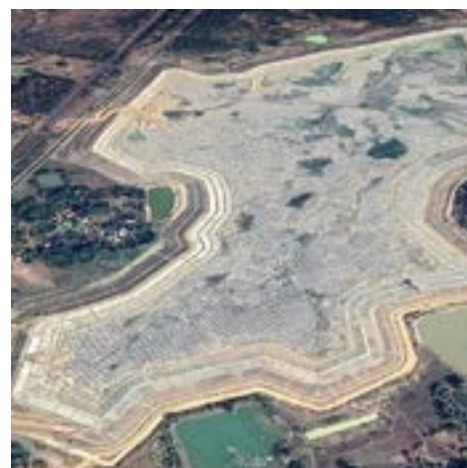
Ash pond with Water Recovery System, Bakreshwar, West Bengal
