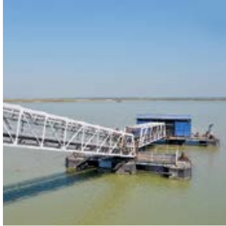
Floating barge intake, Sahibganj, Jharkhand
