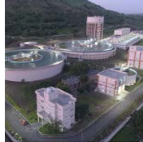
137 MLD Water Treatment Plant at Nashik, Maharashtra
