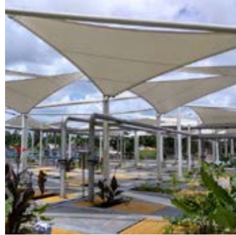
31 MLD Wastewater Treatment Plant, Bhatpara, West Bengal
