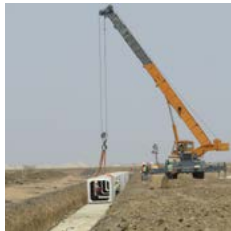
Precast duct laying at Amaravati, Andhra Pradesh
