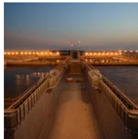
241 MLD Wastewater Treatment Plant, Doha, Qatar
