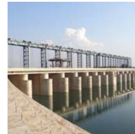
Kharkai Barrage, Jharkhand
