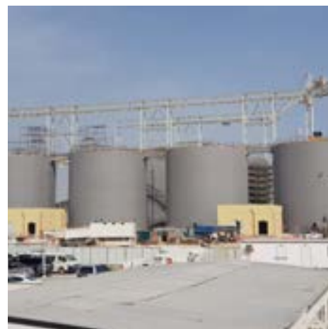
Anaerobic digesters
