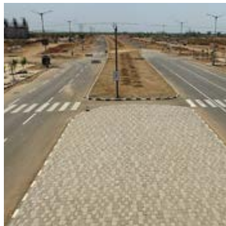
Green-field development at Dholera, Gujarat
