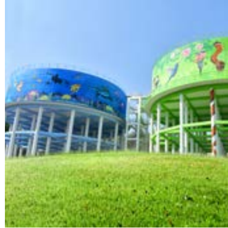
Elevated Storage Reservoir, Pune, Maharashtra
