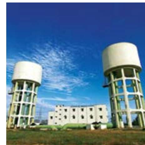
Ali Sagar Lift Irrigation Scheme, Telangana
