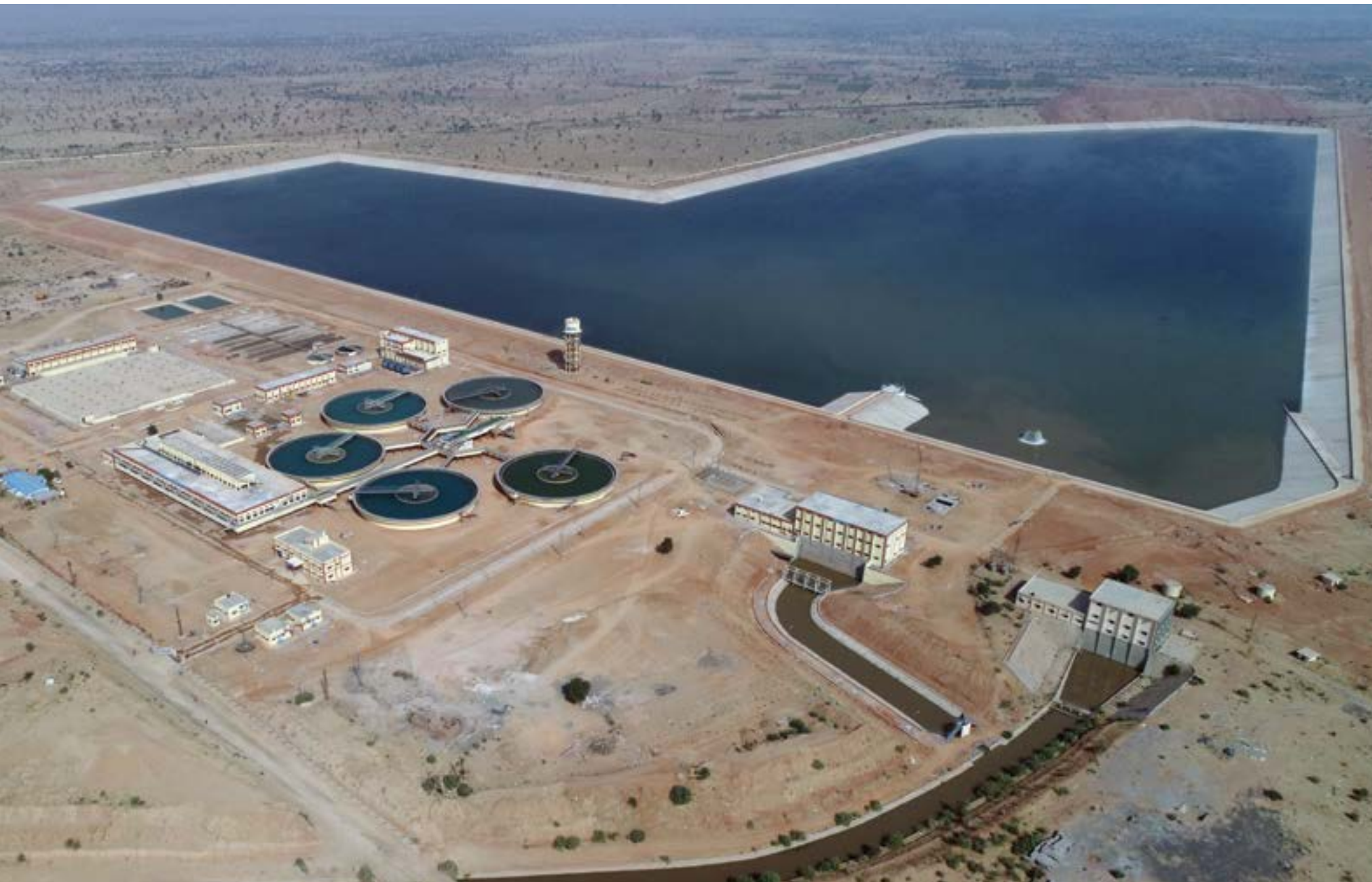
Aerial view of the 250 MLD Water Treatment Plant and 5310 ML Raw Water Reservoir, Nagaur, Rajasthan
