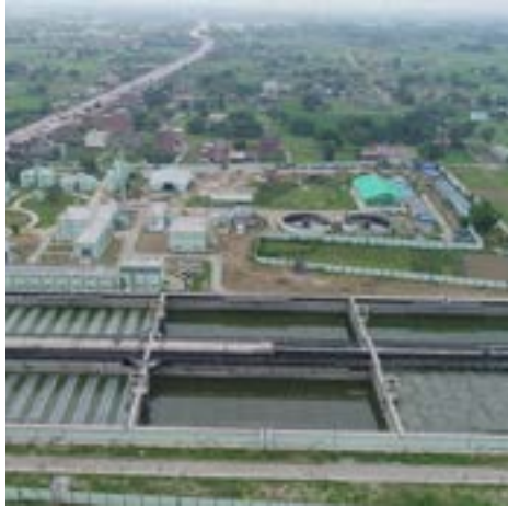
120 MLD Wastewater Treatment Plant, Varanasi, Uttar Pradesh
