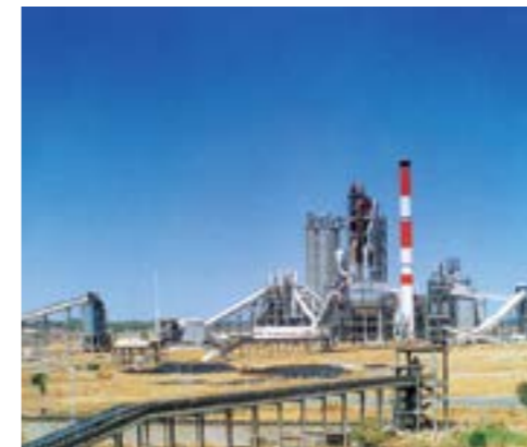
Hirmi cement plant, Raipur
