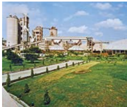
Cement plant at Awarpur, Maharashtra
