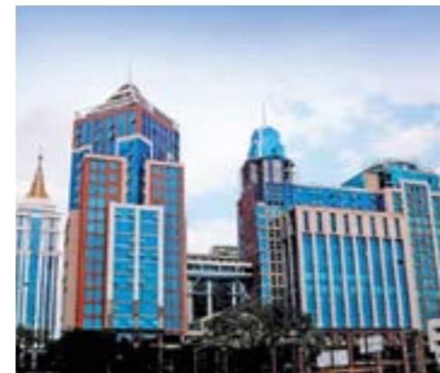
UB Towers, Bengaluru
