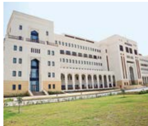
Ministry of Manpower building, Oman
