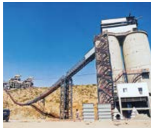
Silos and conveyor at Tadipatri cement plant
