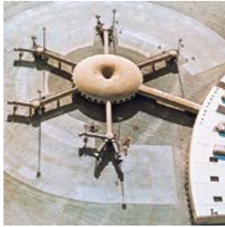
Abu Dhabi International Airport
